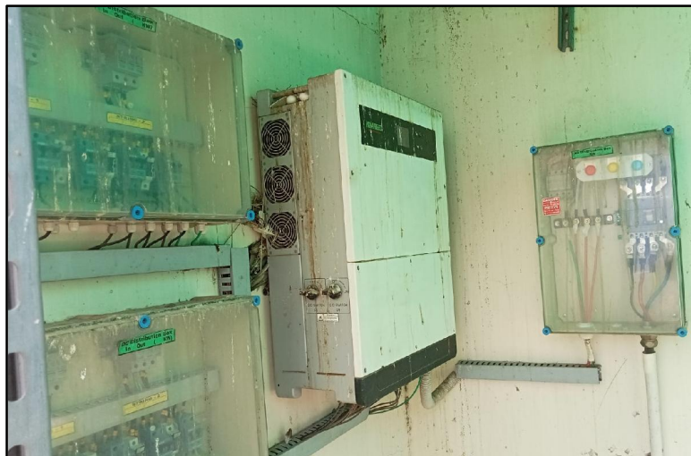
Solar Panels on rooftop
