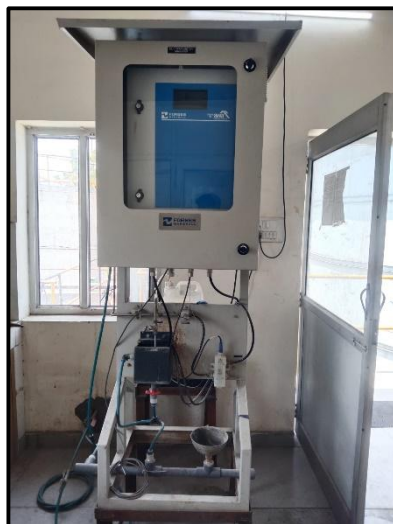
Online Continuous Monitoring System
